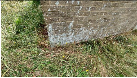
Various minor repairs of brick work.
